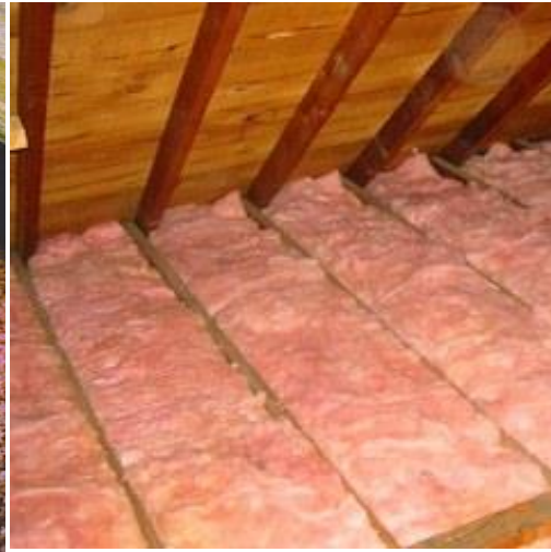
b) Batt insulation
