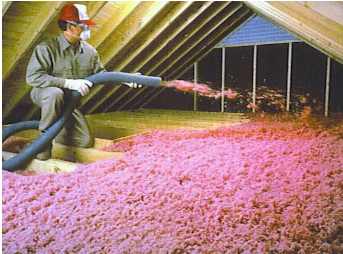
a) Blow-in insulation
